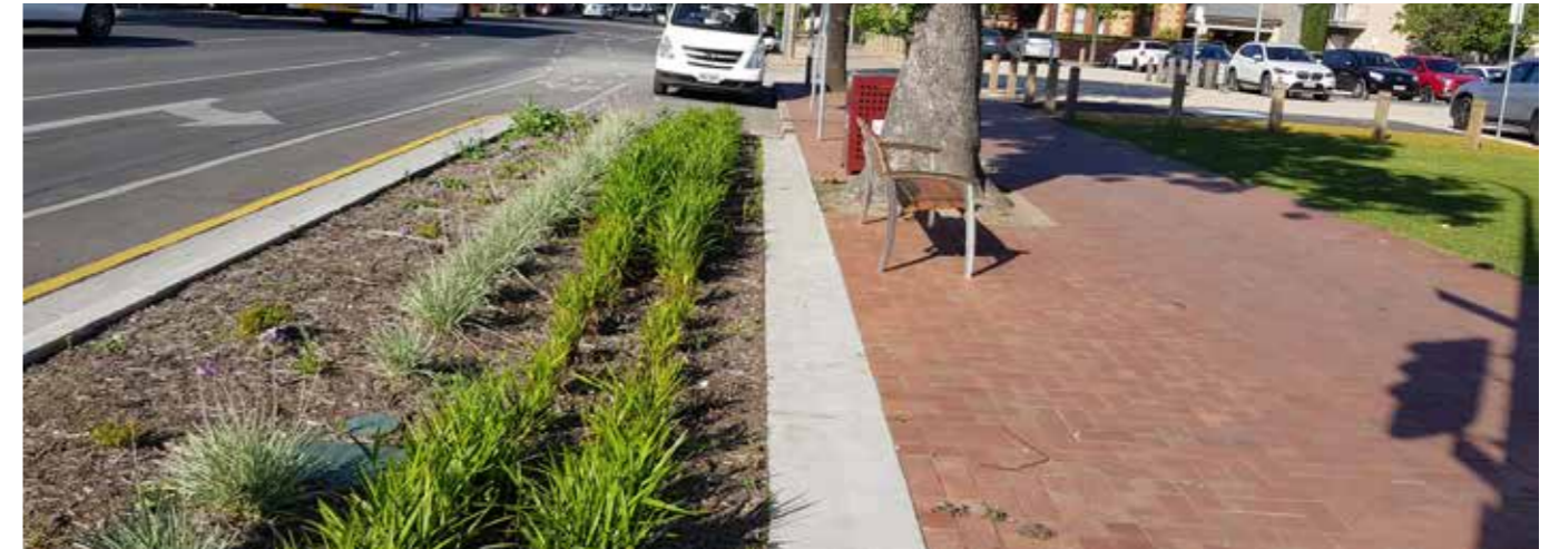
2018 upgrade of Tynte Street intersection with increased greening and upgrades to kerb, footpath and gutter
