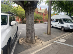
Tree pit too small stobie pole in middle of car parks
