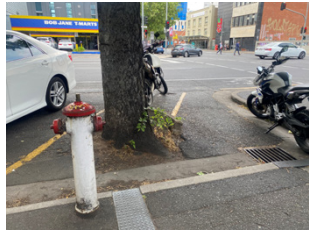
Tree pit small for tree growth in poor condition
