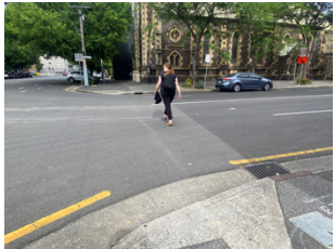
Unsafe crossing across four lane vehicular traffic
