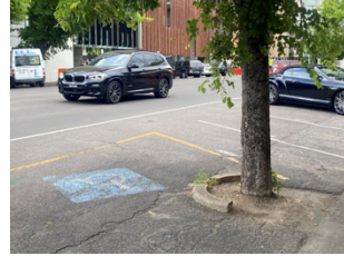
Confusing accessible car park line marking and tree pit
