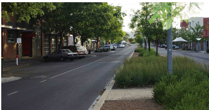
Median with trees planting, shrubs and informal crossing points
