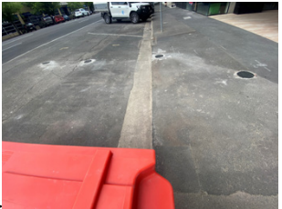
Construction site removed trees to be reinstated by agreement
