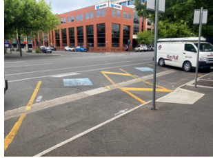
Wide road, hard for wheelchair across it safely
