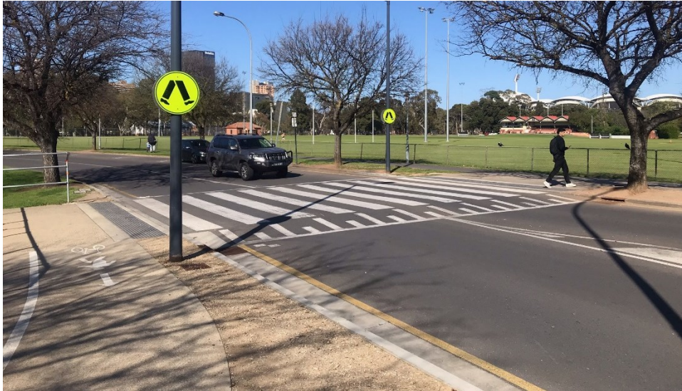
Figure 24 A Wombat (Raised Zebra) Crossing on War Memorial Drive at the Frome Road Roundabout
