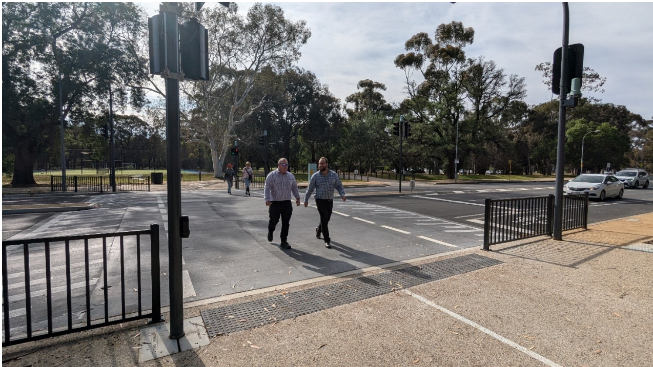
Figure 16 People Crossing on a Raised Safety Platform as Part of a Bicycle Pedestrian Actuated Crossing (BPAC)
