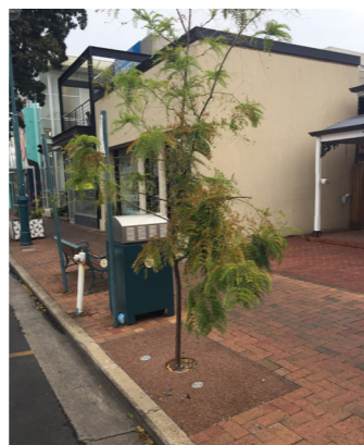
Recent tree planting with bonded aggregate and tree vents
