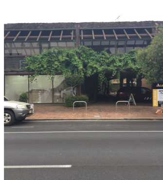
Existing greening to pergola/ arbour structure
