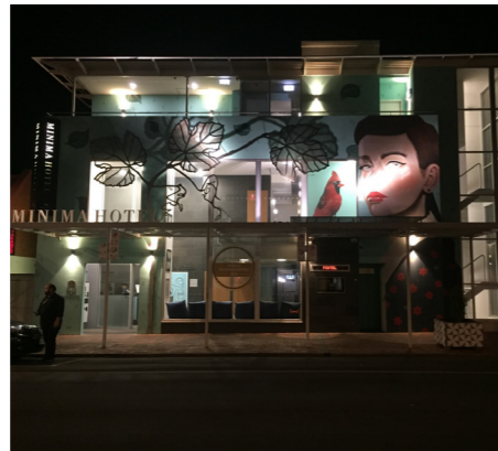
Building and artwork lighting with room for improvement.
